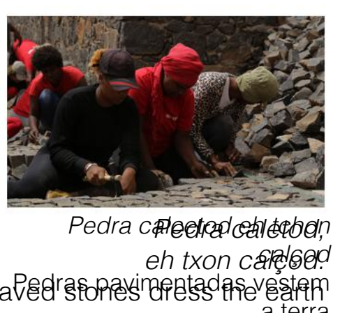
Start of the works
